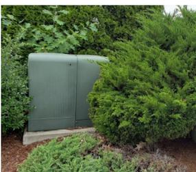
When our line workers or engineers have to service transformers that are surrounded by shrubs, we must first remove the overgrown vegetation from the easement area.
